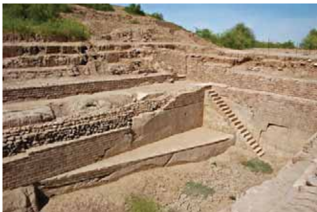
The Water Tank at Dholavira
