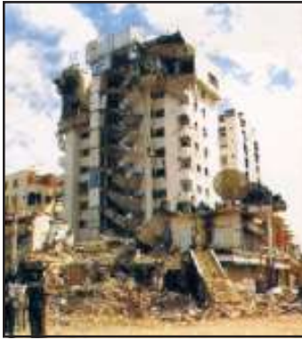
Fig. 3.3a: Destruction caused by an Earthquake in Gujarat
