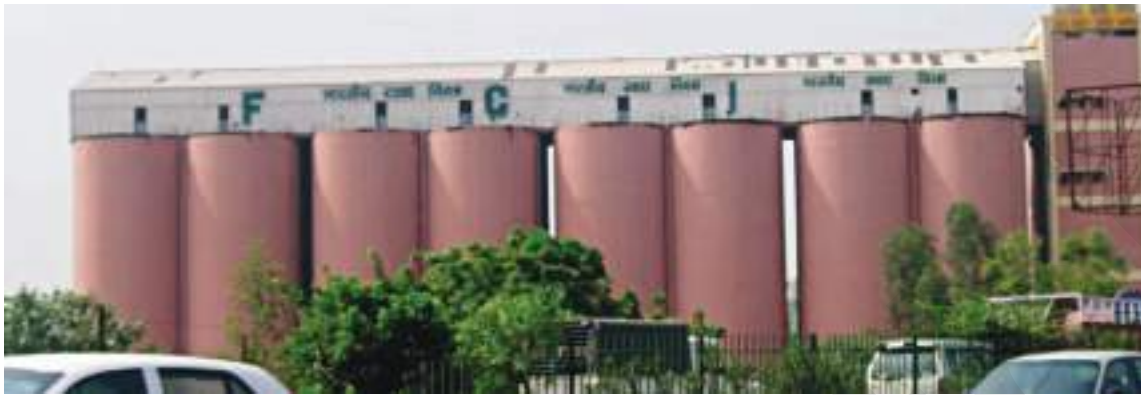
Fig. 1.10 (a) : Silos for storage of grains
