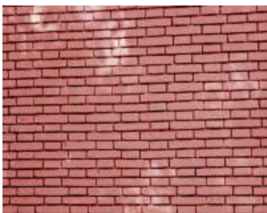
(a) Brick wall
