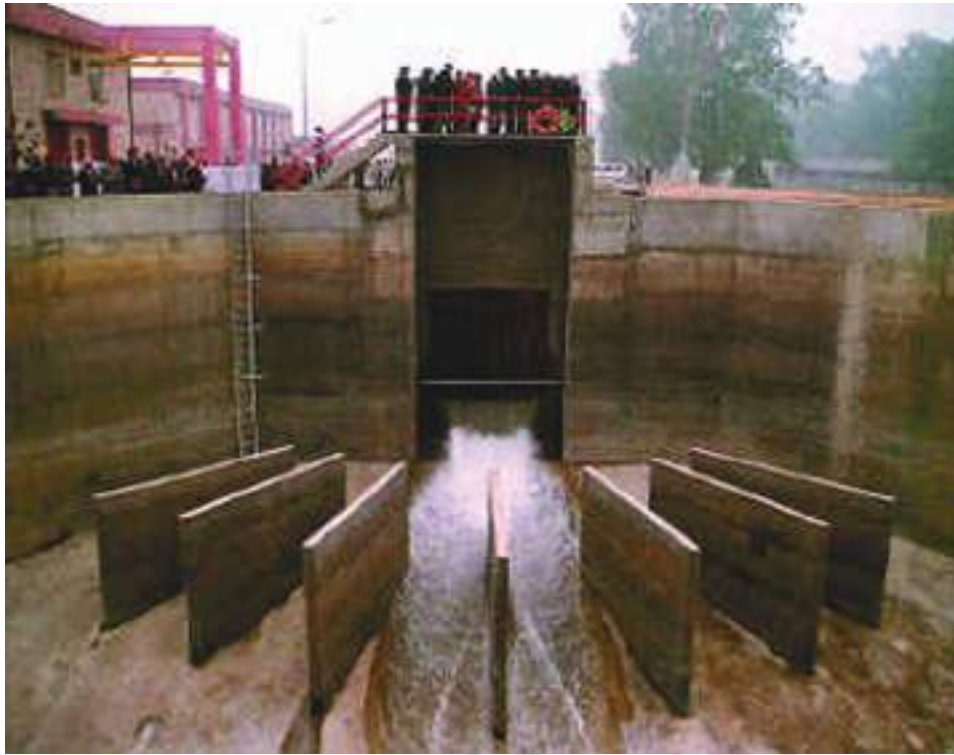
Fig. 18.10 : Water treatment plant
