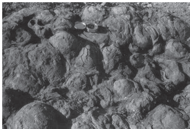
Fig.5.3 : Exfoliation (Flaking) and granular disintegration
