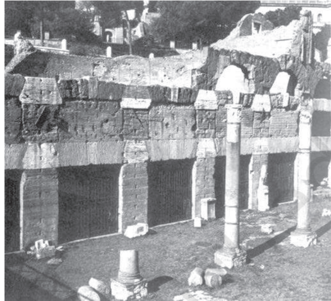
Shops in Forum Julium, Rome. This piazza with columns was built after 51 BCE, to enlarge the older Roman Forum.
