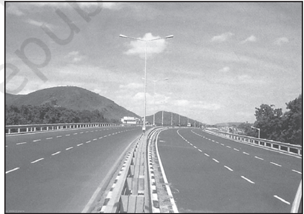
Fig. 7.3 : Dharmavaram Tuni National Highway, India
