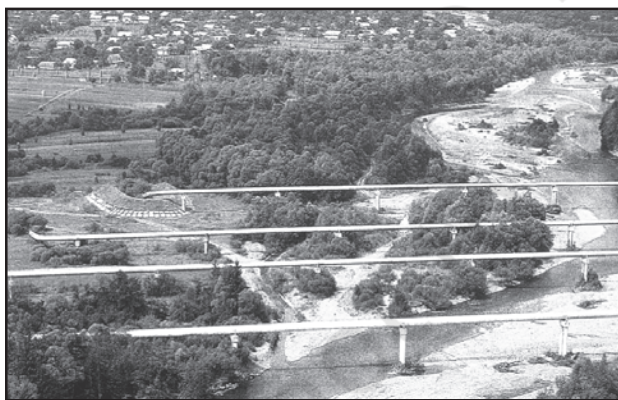
Fig. 7.17: Pipelines transporting natural gas in Ukraine
