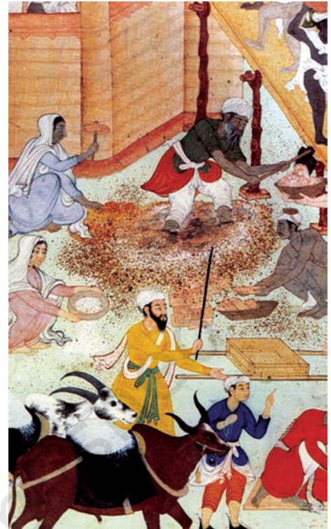
Fig. 8.8 a The construction of Fatehpur Sikri – women crushing stones
