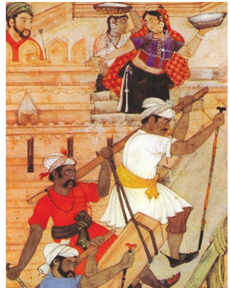
Fig. 8.8 b Women carrying loads Migrant women from neighbouring villages often worked at such construction sites.
