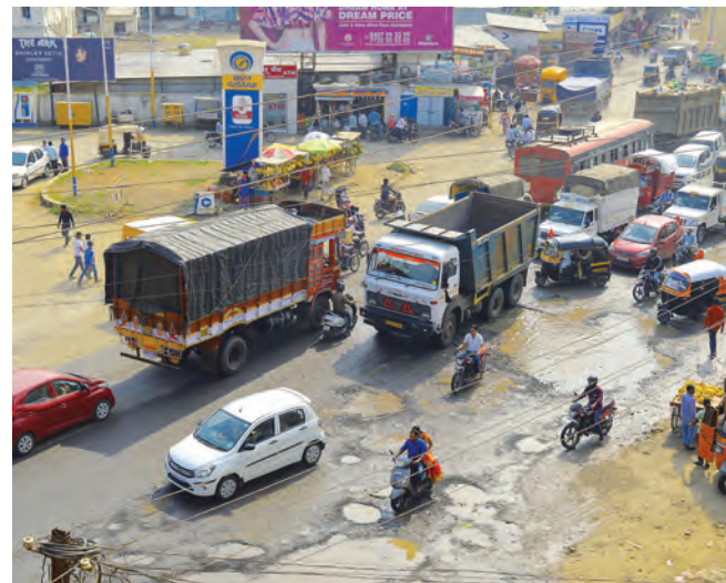
Fig. 7.27. Potholes on the roads
