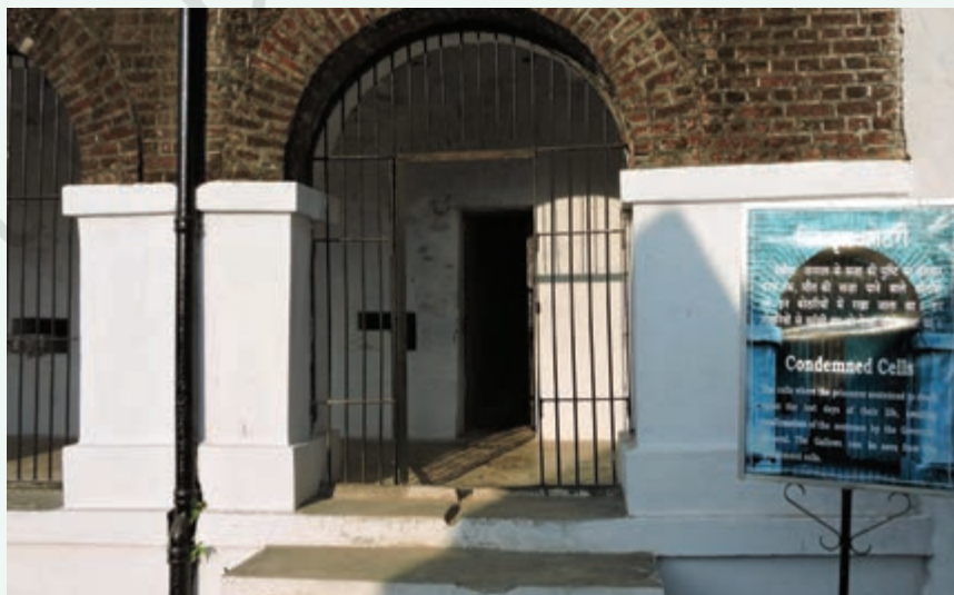
Fig. 2.20. In the Cellular Jail, prisoners condemned to death were kept in this separate cell before being hanged.
