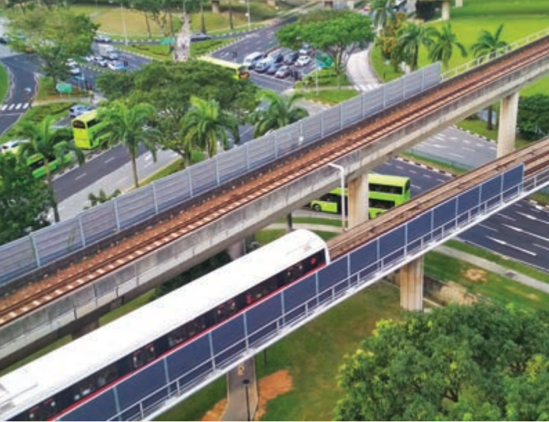
Fig. 7.26. Mass Rapid Transit, a railway system connecting the main parts of the city
